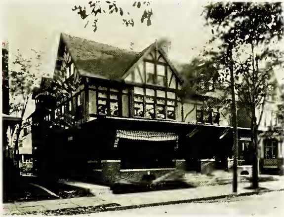
Residence of E. W. Marple South Franklin Street
